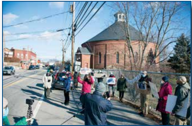
At this time last year, demo of the last-of-its kind 1888 Concord Gasholder seemed like a real possibility. Owner Liberty Utilities, the City of Concord and the Preservation Alliance, working together, identified funds pledged for emergency stabilization, attracting widespread public support and creating a sense of opportunity ahead.
