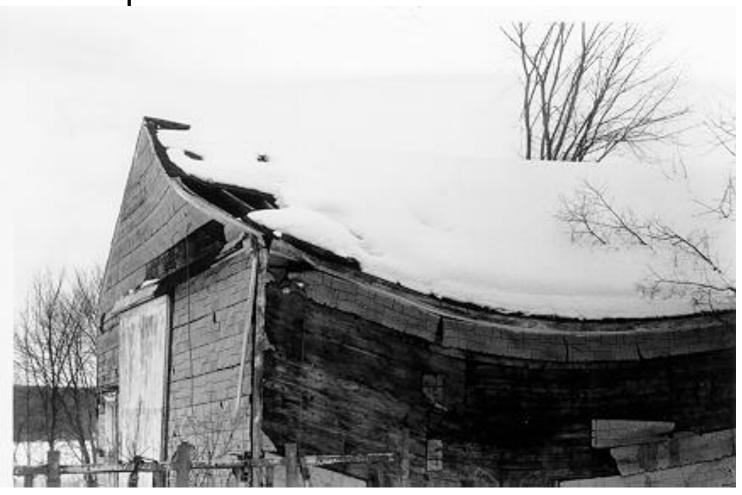
4.) Fix crumbling foundations, as they are the key to maintaining a square and plumb building.
